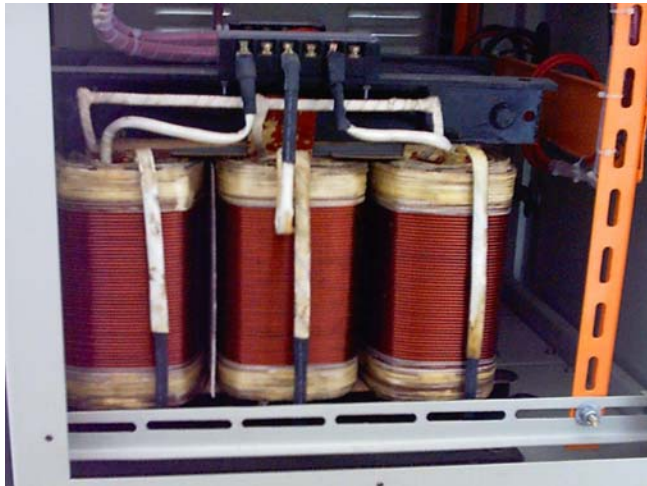
3 Phase Main Isolated Transformer.
